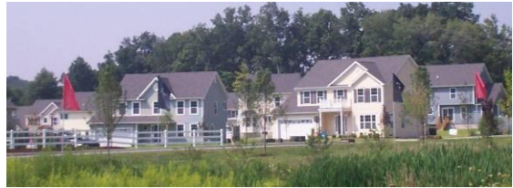
New construction in Beekman.
