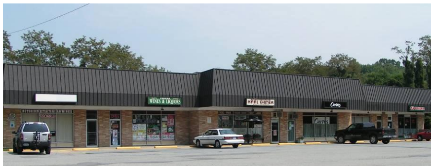
Commercial Plaza located on Route 55.
