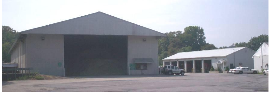
Beekman Highway Garage and Salt Shed.
